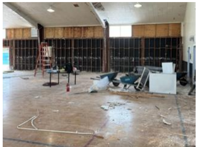
The north wall is being demolished and will extend out 12 feet!
