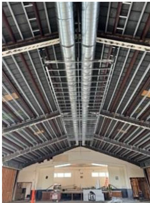
New AC/Heating ducts and fire sprinkler systems are being installed in the ceiling.
